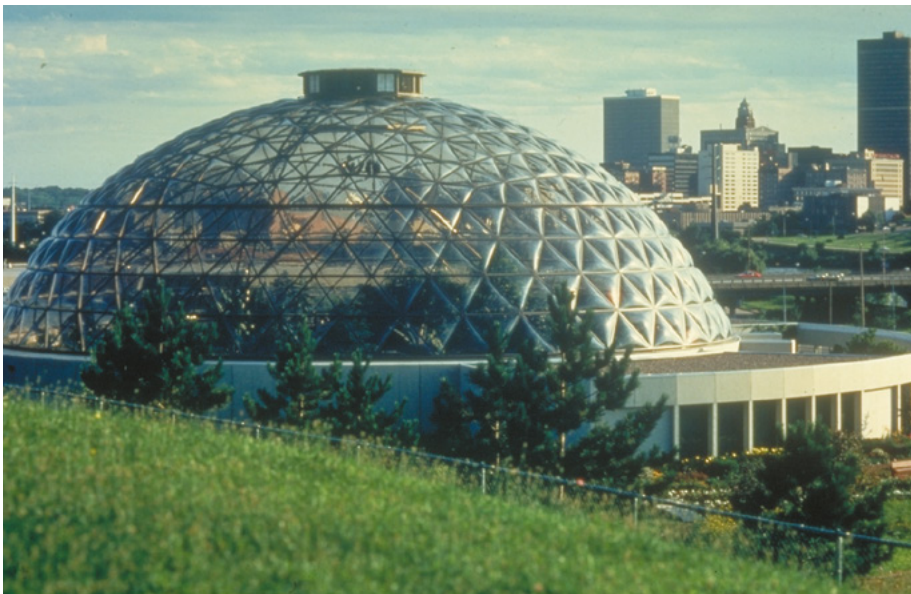
Botanical gardens, Des Moines, Iowa, USA, 46m dome structure.
