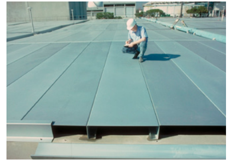
Aluminium flat covers for sedimentation bassins.
