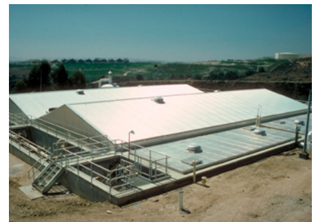
Waste water treatment plant, USA, batch reactor, truss roofs and aerobic digesters.
