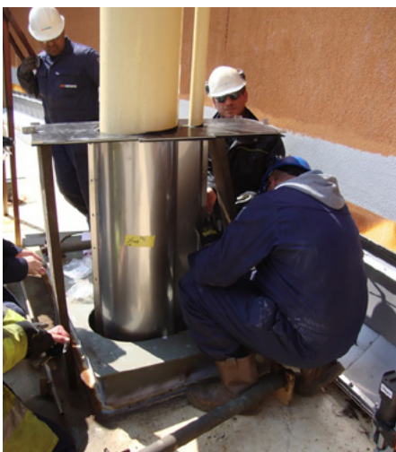
Gauge pole sleeve during installation.
