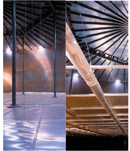
Cable suspended IFR, no legs, top and bottom view.
