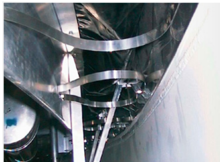
Liquid mounted shoe plate seal on skin and pontoon IFR.
