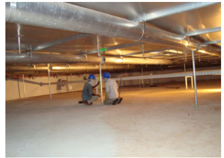
IFR's and domes make a great alternative for replacing a corroded steel roof.
