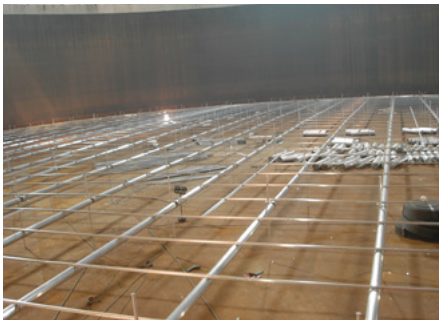
Skin and pontoon IFR under construction, 70m diameter.
