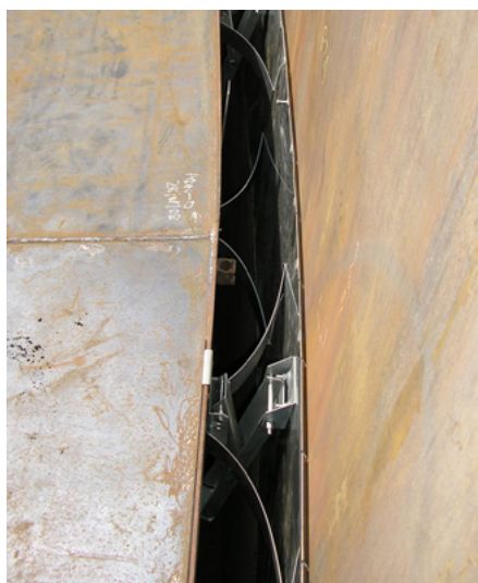
CTS1 scissor shoe plate seal, top view during installation.
