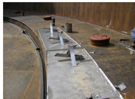
CTS1 scissor type shoe plate seal with energised hangers, ready to be fitted.
