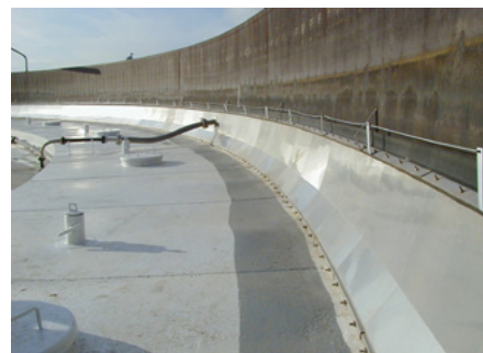
CTS20L secondary seal with direct foam injection.
