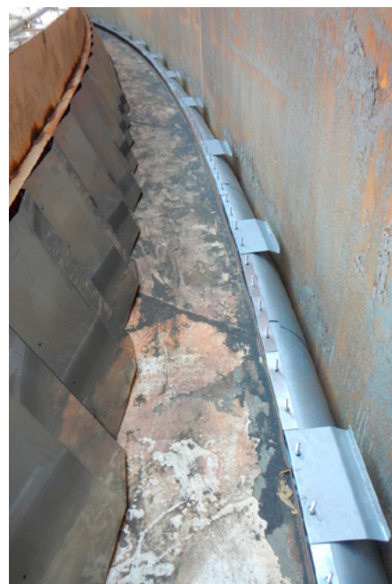
CTS30 seal during installation, top view.
